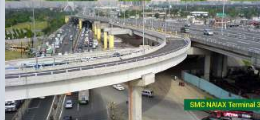
Cavite-Laguna Expressway (CALAX)
